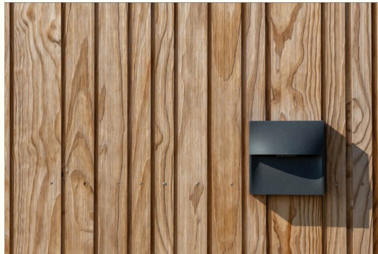
Imbue Cladding, Sydjylland, Denmark. Installed 2024.
