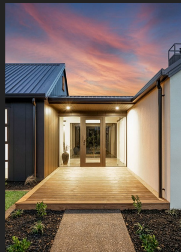
Imbue Decking, Whatawhata, New Zealand. Installed 2022.
